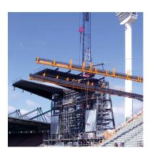
The 2006 Commonwealth Games in Melbourne were a fitting debut for the magnificent new Northern Stand at the Melbourne Cricket Ground (MCG). The three year redevelopment project valued at \$434 million used approximately 1000 tonnes of Orrcon Steel's Smart Steel Hollow Sections in the support columns, seating framework and roof structure.
