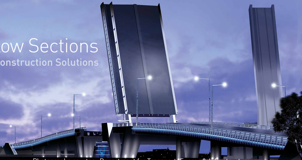
Photographs courtesy Department for Transport, Energy & Infrastructure
